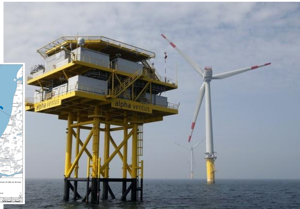
Wind farm transformer station
